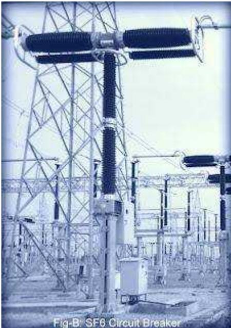
Fig-B: SF<sub>6</sub> Circuit Breaker
